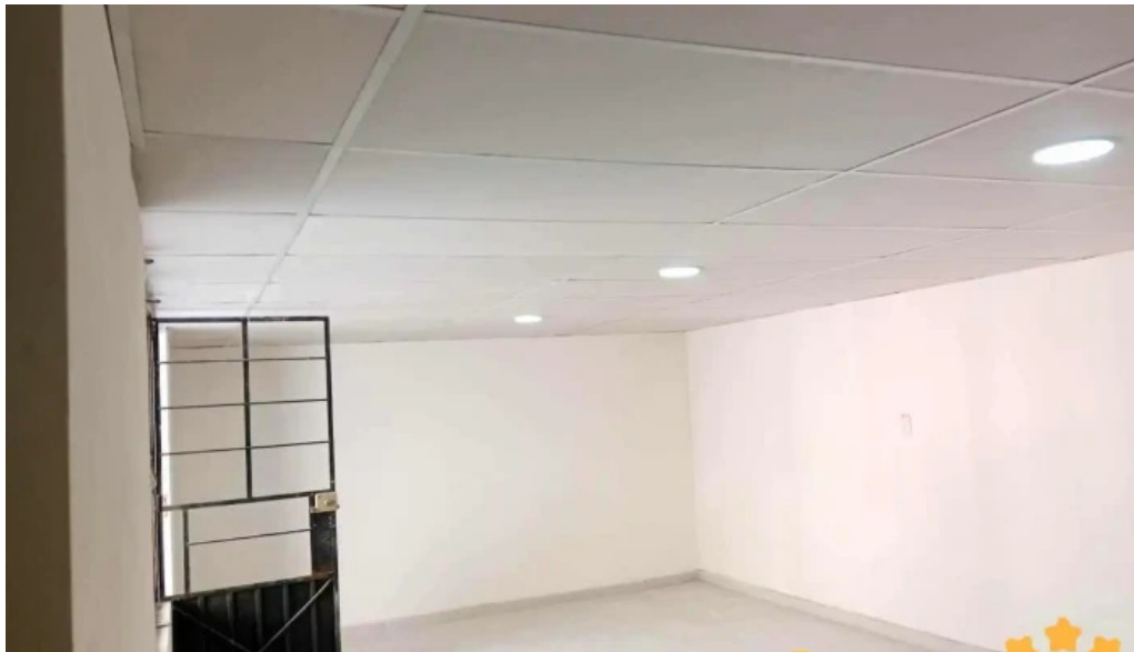
Instalaciones electricas electricista blean electricity interior
