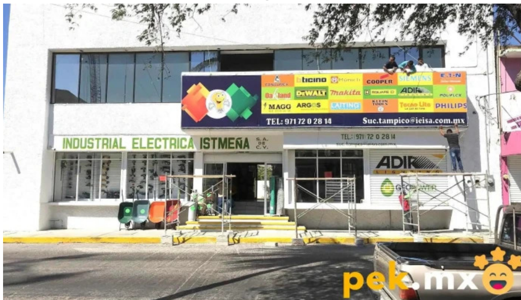
Industrial electrica istmena salina cruz
